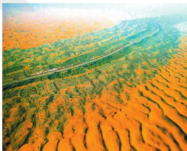
Figure 1 Prevention and control project for blown-sand hazard in Shapotou section of Baotou-Lanzhou Railway
